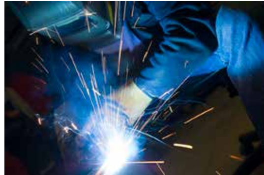
On-Site Coded Welders
